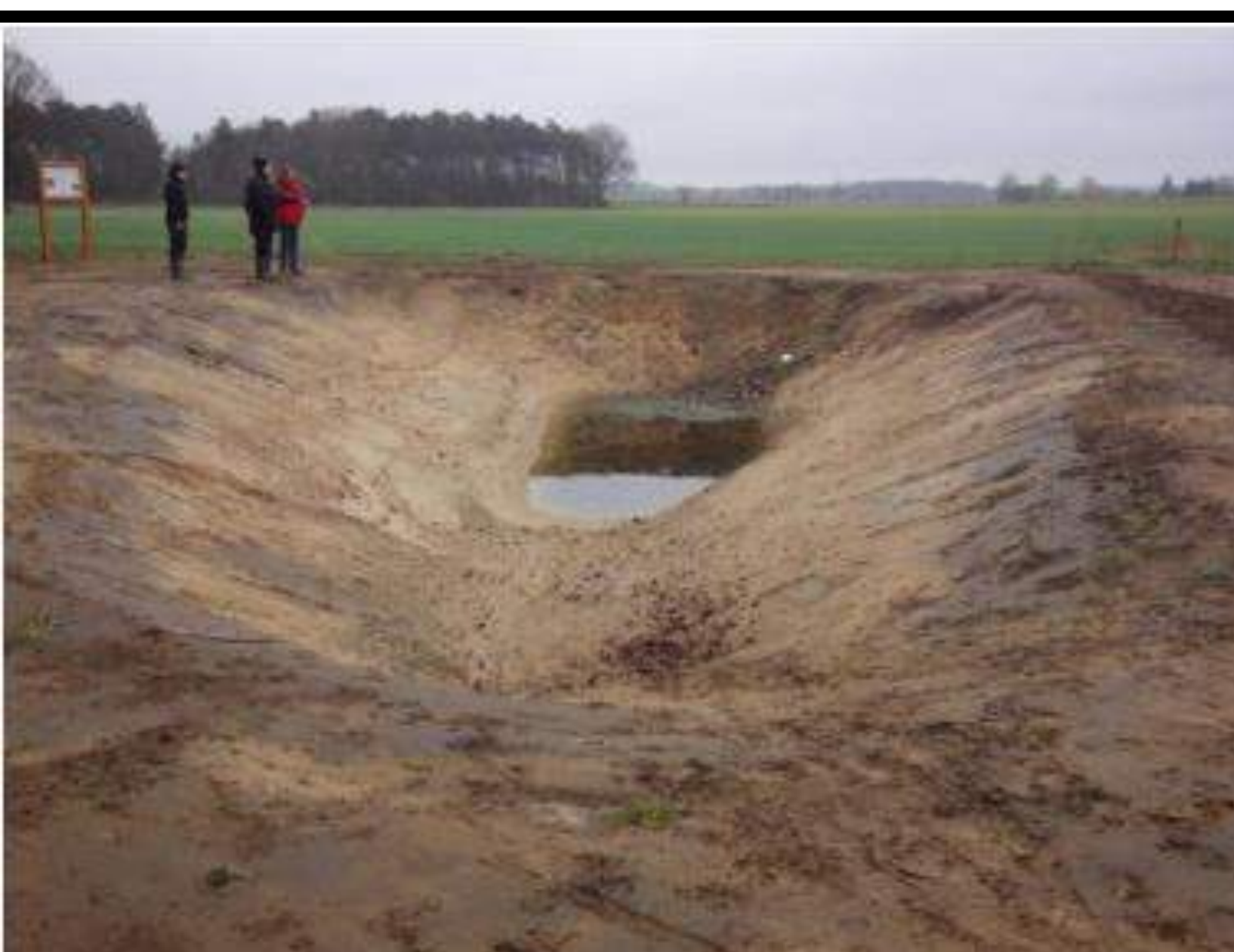
Construction of alternative collection drain from before leading into a creek and now to the newly created seepage pond in 2010/11. The pond is now completely ingrown with shrubs.
