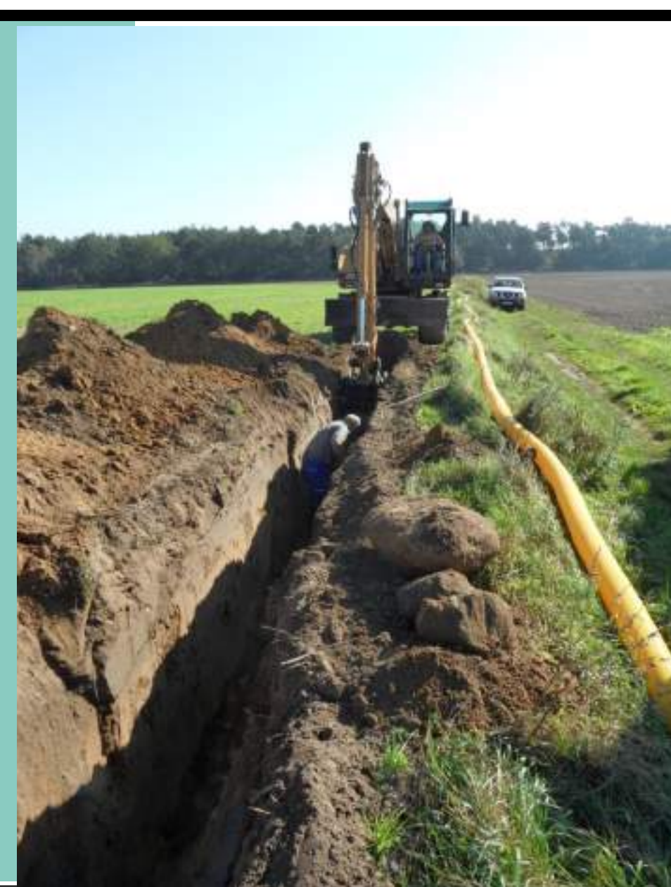
Construction of alternative collection drain from before leading into a creek and now to the newly created seepage pond in 2010/11. The pond is now completely ingrown with shrubs.
